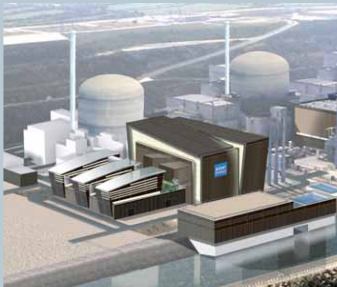
In October 2004, the French utility Electricité de France (EDF) selected Flamanville in Normandy as the site for the first EPR in France (on the left in this photo montage).
