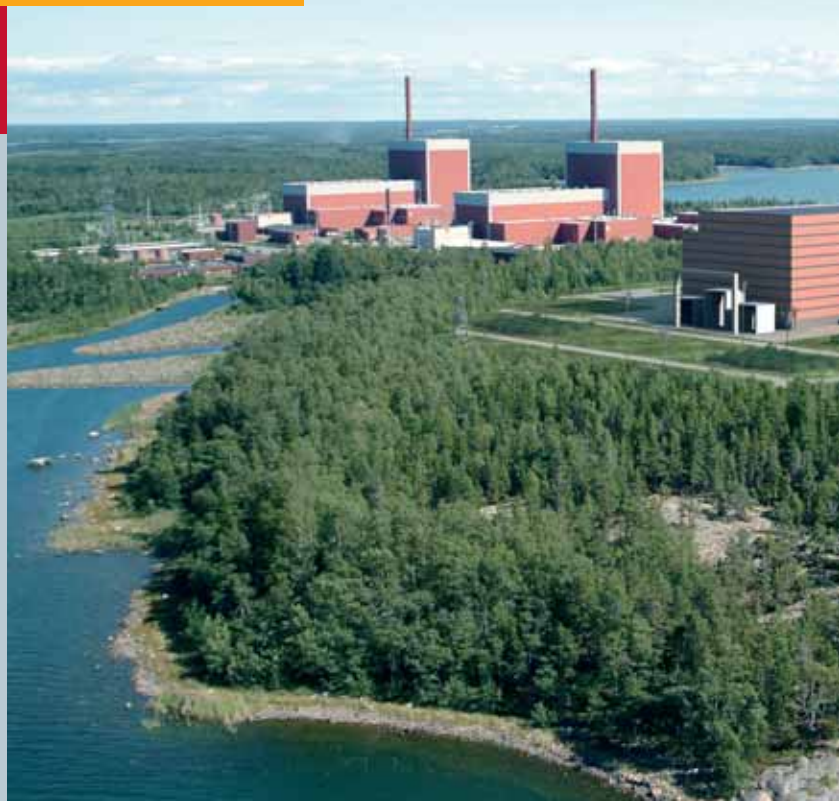
The first EPR (on the right in this photo montage) is being built for the Finnish utility Teollisuuden Voima Oy (TVO) at Olkiluoto in Western Finland. Commercial operation is scheduled to start in 2009.
